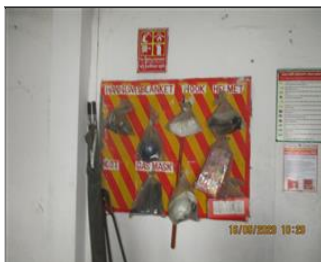
Photo of fire safety equipment Firefighting equipment.JPG
