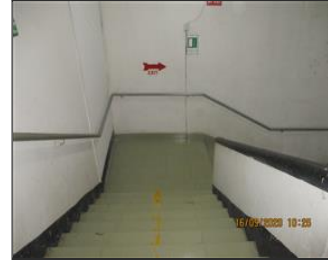
Photo of the inside of the main production hall Stair case.JPG
